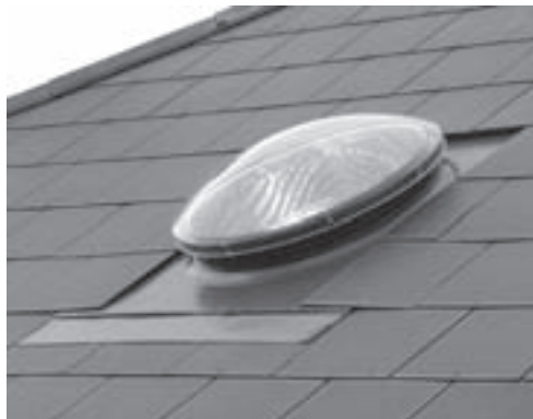
Sky Tunnel - Slate Flashing
